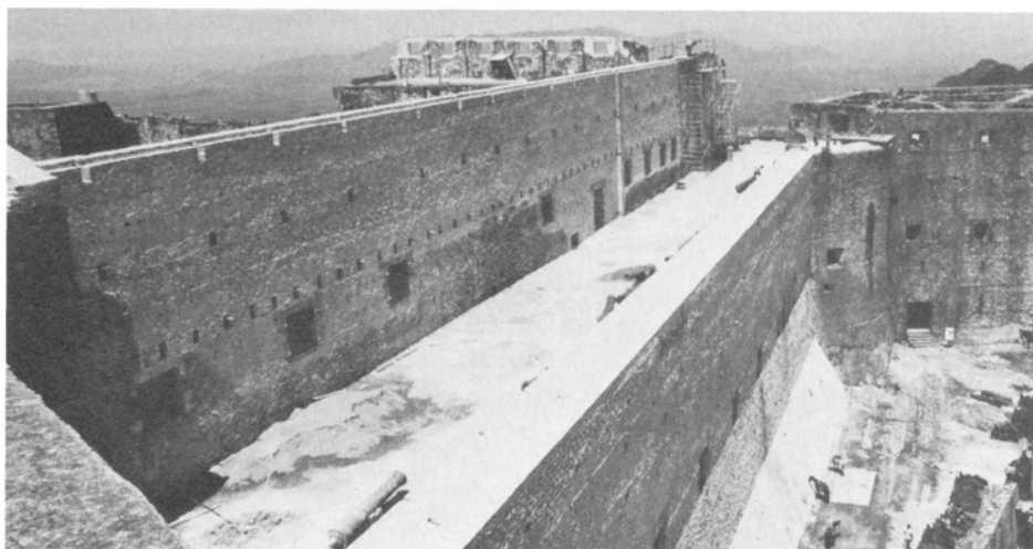
Partial demolition, above, and restoration, below, of a wall on the Royal Battery at the Citadelle. The Governor's Palace is beyond the battery in these pictures. Holes in the wall are anchor points for trusses that
