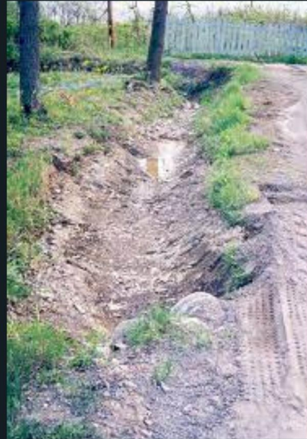
An eroded roadside ditch. Cornell Local Roads Program
