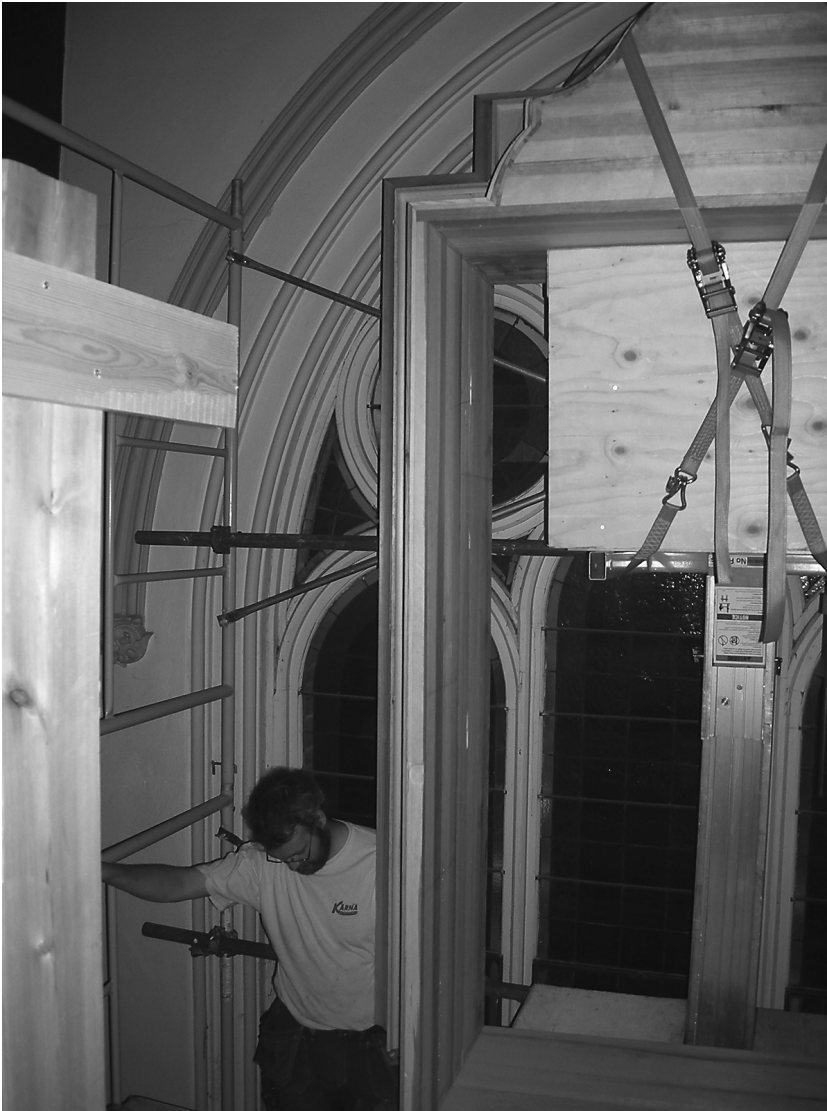
Figure 5 Raising the left pedal tower in Rochester. Photo: GOArt archive.
