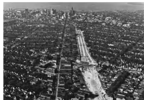
Figure 4. Construction of the Kensington Expressway, one of the major physical dividers of the East Side of Buffalo.
